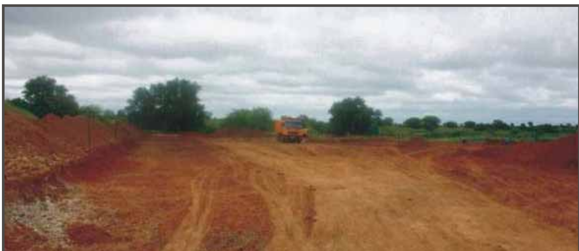
Commencement of excavation and rehabilitation work
