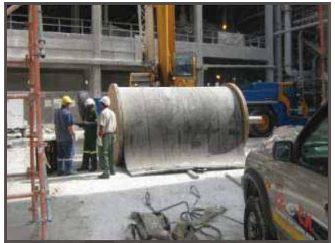
Main Belt replacement of Belt Filter-2
