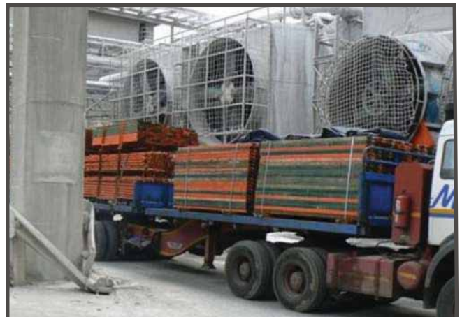
Approximately 400MT of scaffolding was brought in for the shut down
