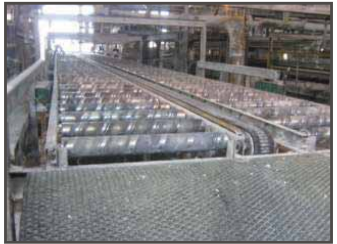
Belt Filter-2 to receive new belt
