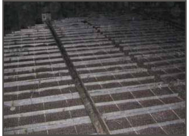
Demister pads replacement in the Drying Tower
