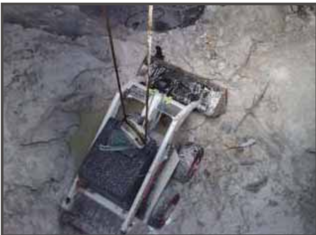
Bobcat being placed by crane inside Reactor for cleaning
