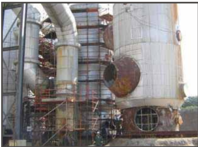
Cold Heat Exchanger replacement
